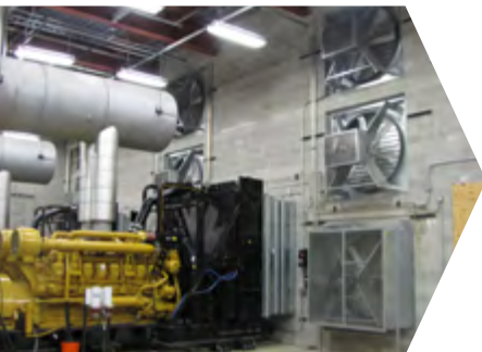
Generator Room Exhaust
