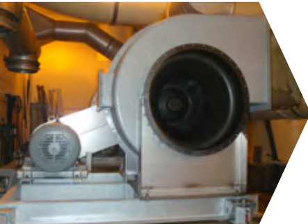
Odor Control Waste Water Treatment
