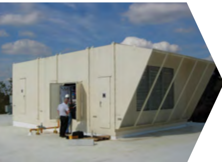
Heavy Industrial Supply Air
