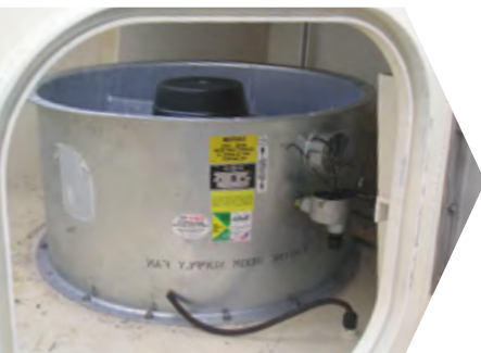
Engine Room Supply Fan (Marine)
