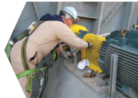
Coupling Alignment
