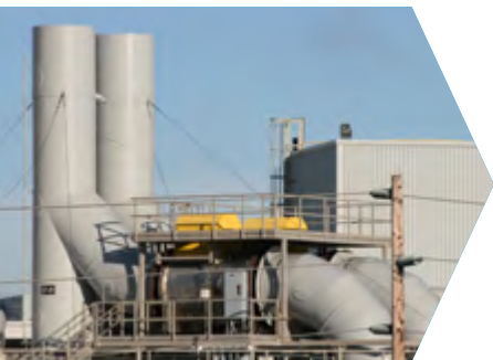
Paint Booth Exhaust
