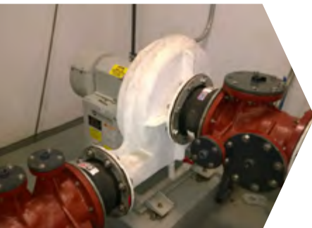
Odor Control Water Treatment
